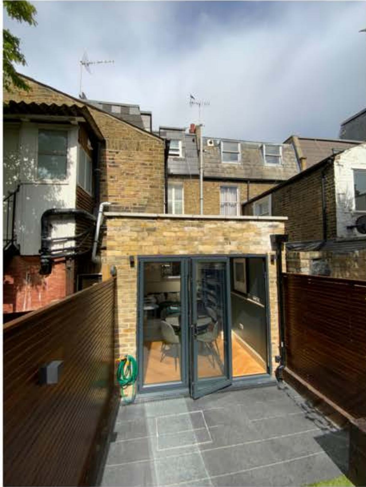
01 Sliders leading out to the garden area. London stocks used to seamlessly tie this extension into the existing build.
