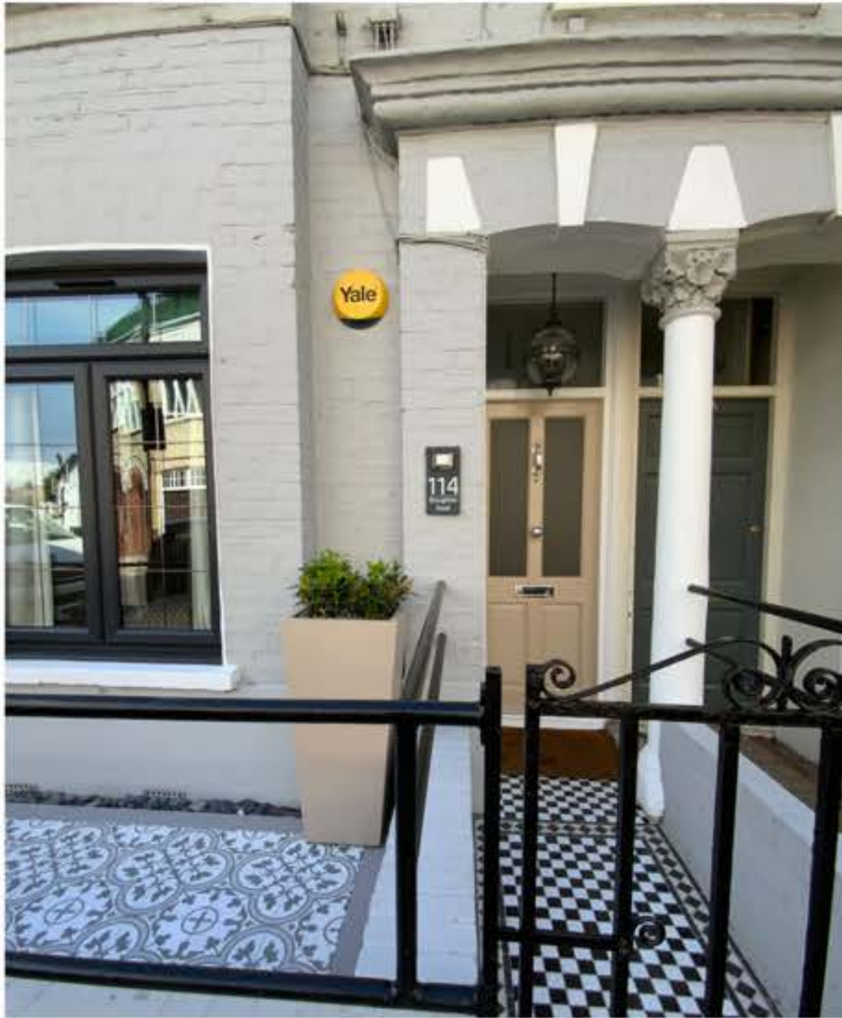
01 Completely refurbished front of the property.
